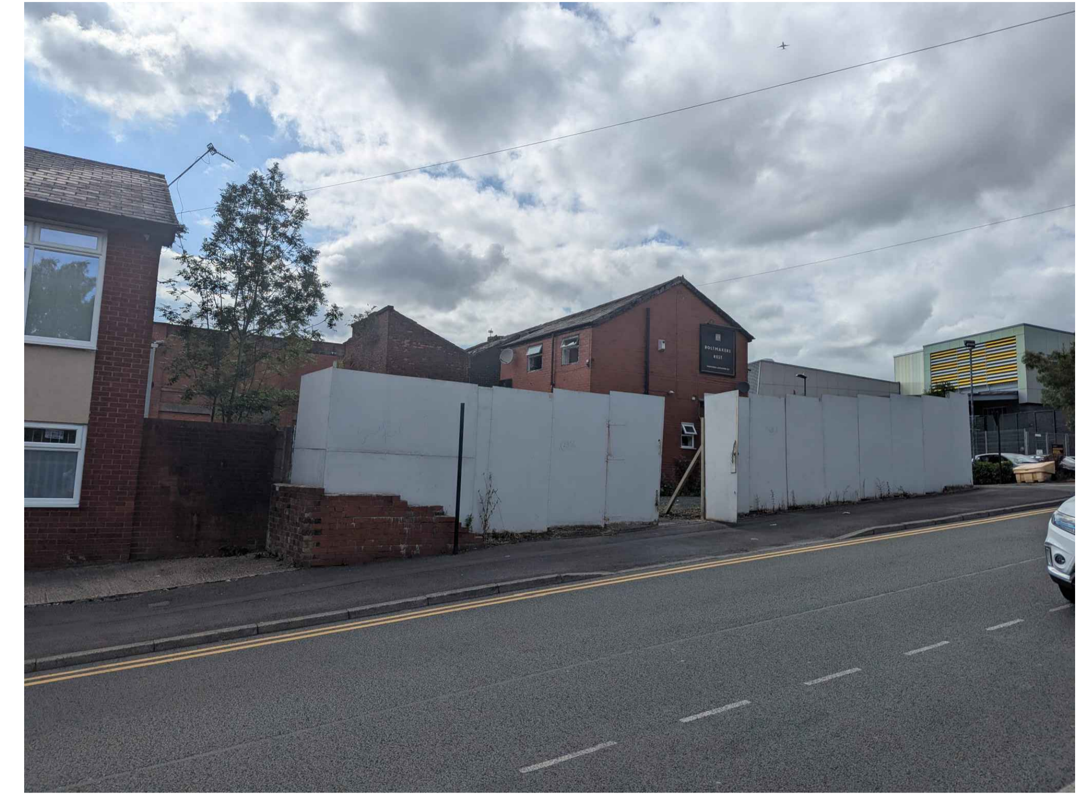
CURRENT BOUNDARY WALL AND ACCESS FROM HORSEDEGE STREET WALL TO BE MADE GOOD AND SECURITY GATE AND FENCING TO BE ADDED
